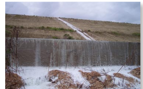
Phosphoric Acid spilling from phosphogypsum stack near Houston, TX.
